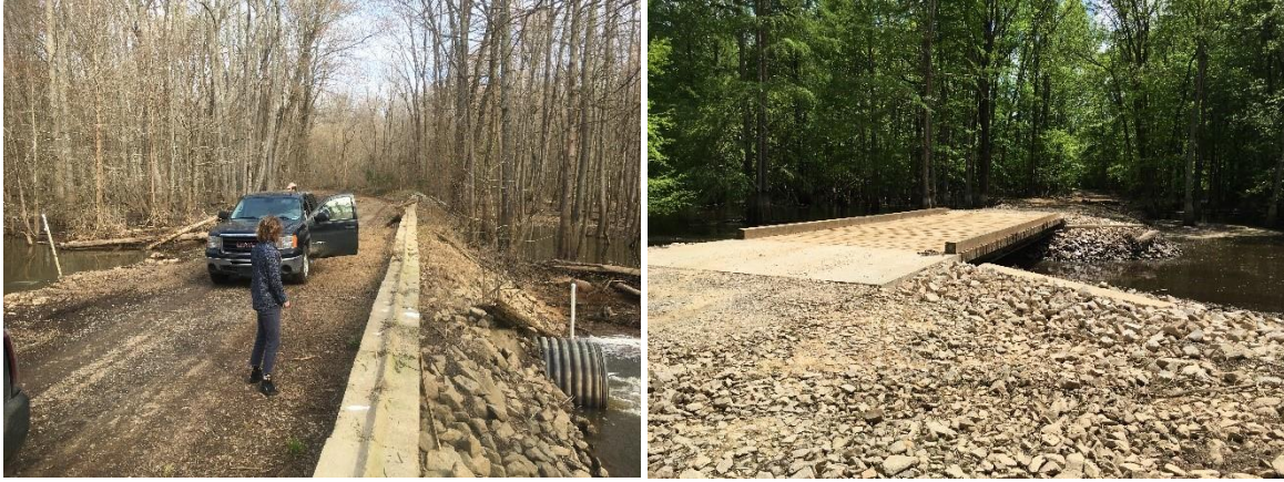
Figure C 46- Phase 2 crossing with culvert (before, left) and bridge (after, right). Credit: Aaron McCall/ TNC.
