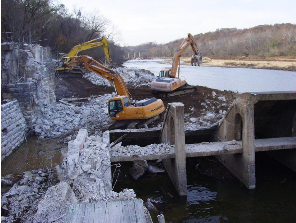
Figure C 41 – Mechanical removal of the remaining structural pieces of the Embrey Dam. Credit: Alan Weaver/ VADWR.
