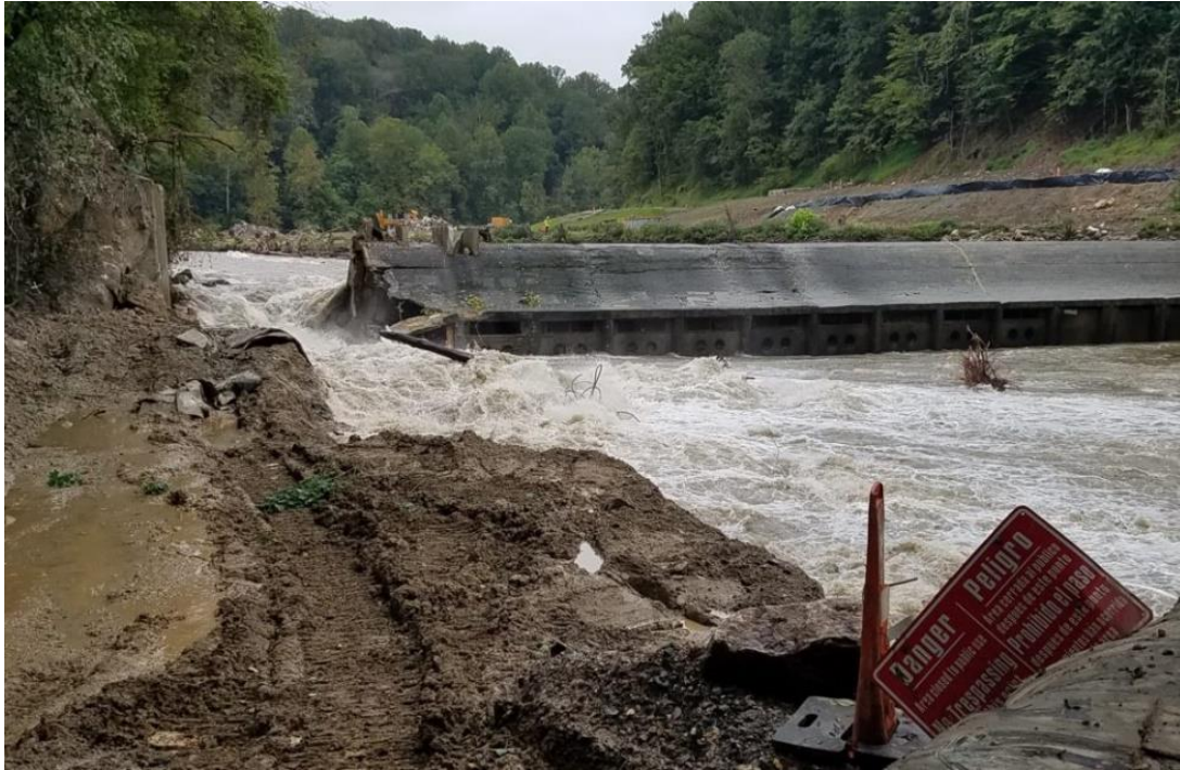
Figure C 35 - Bloede Dam after initial breaching. Credit: Jim Thompson/ MDNR.
