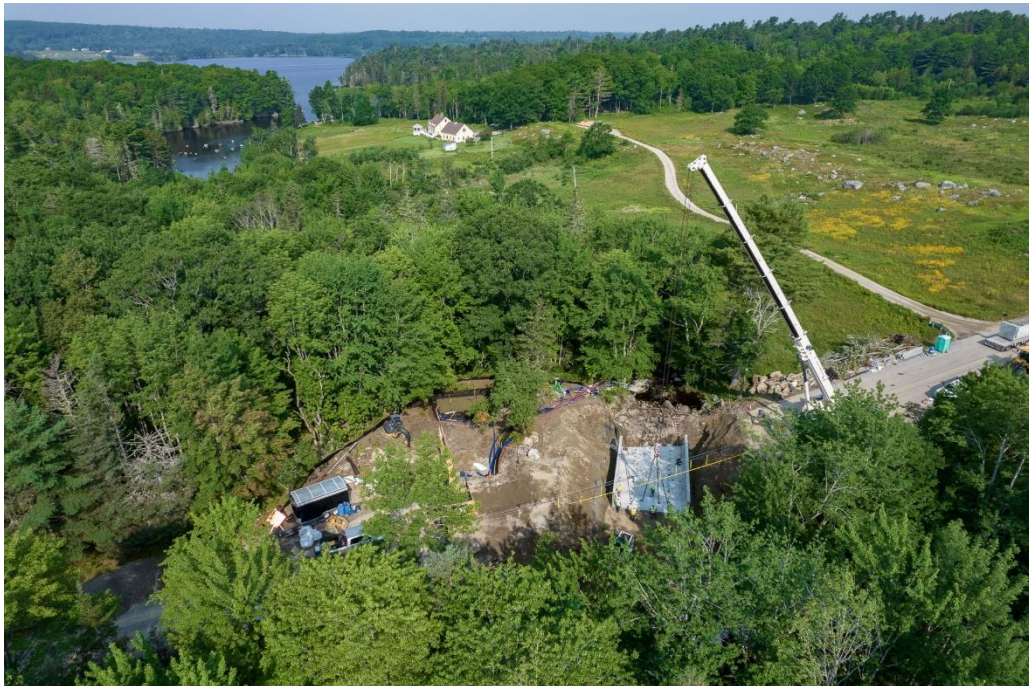
Figure C 5 – Aerial view (perpendicular to road) of the construction site for the installation of a large box culvert on Snow’s Brook. Credit: Ken Woisard Photography/ MCHT.
