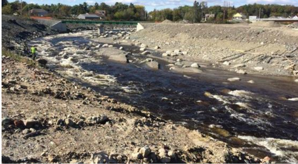
Figure 7 – Howland Dam bypass nature-like fishway on the Piscataquis River in Howland, ME. Credit: NOAA Fisheries.
