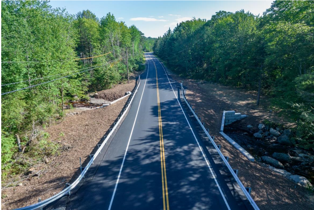
Figure C 6 – Aerial view of fully installed box culvert on Snow's Brook. Credit: Ken Woisard Photography/ MCHT.
