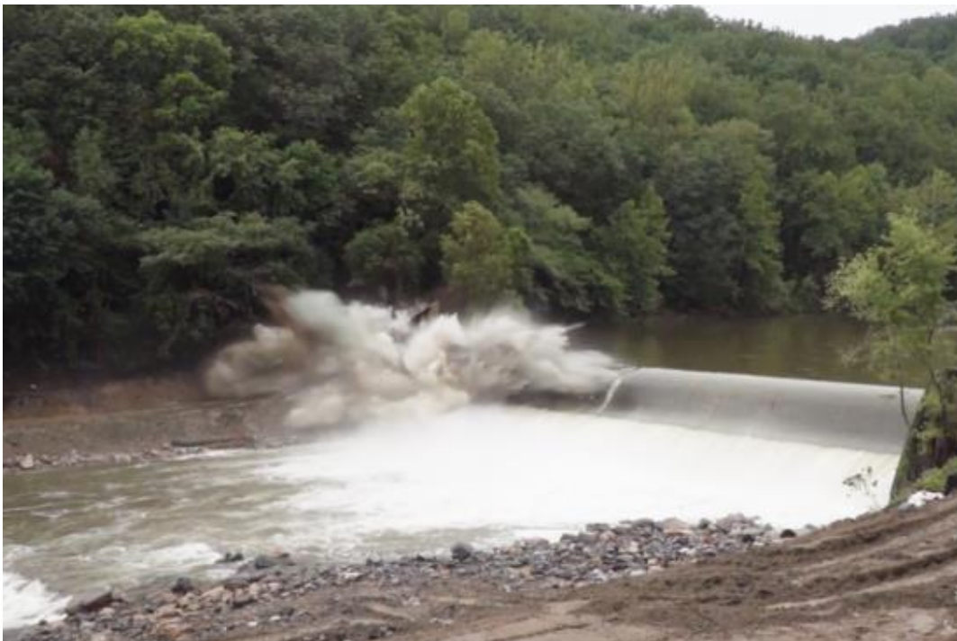
Figure C 34 - Initial Breaching of the Bloede Dam via explosives Credit: Elevate Media, Inc. and MDNR.
