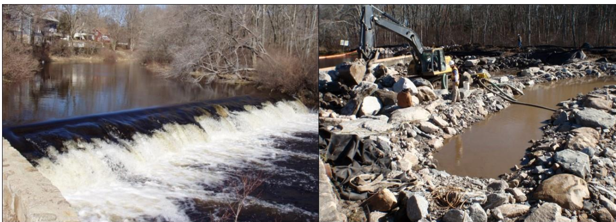
Figure C 20 – Kenyon Mill Dam, pre-removal (left – 2010) and NLF under construction (right – 2013). Credit: NOAA Fisheries.
