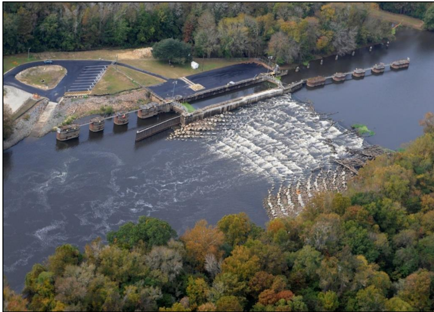
Figure C 50 – NLF installed in place of the Lock and Dam #1 on the Cape Fear River, NC completed in 2012. Credit: USACE.
