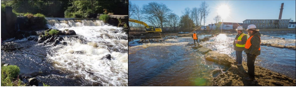
Figure C 22 – Bradford Dyeing Dam pre-removal (left) and installation of NLFs (right) in 2017. Credit: NOAA Fisheries (left) and Ayla Fox/TNC (right).
