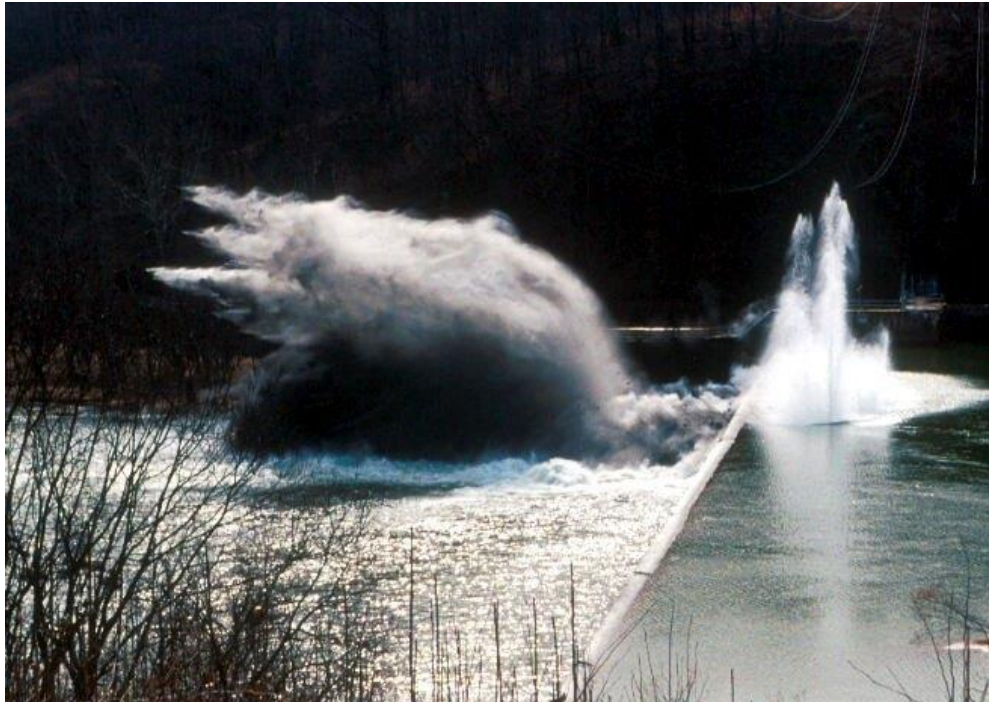
Figure C 39 – The second explosion set off during the demolition day event to breach the Embrey Dam. Credit: VADWR.
